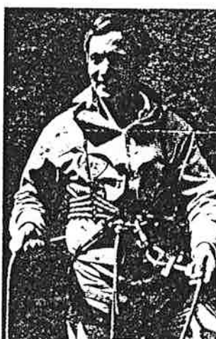
Brake stage Ia: plate and one carabiner + body belay ca. 730 lbs.
